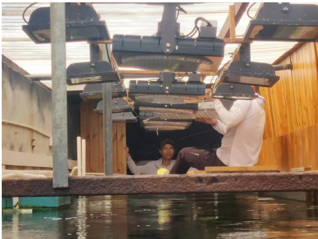
电工在加装十米缸 LED 灯
